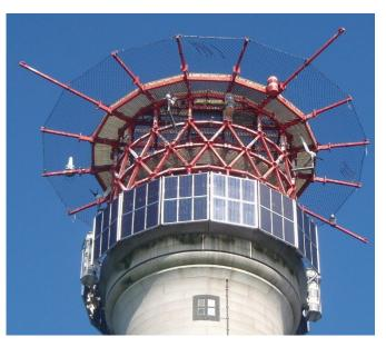
Figure 6 Smalls Lighthouse Hybrid Power System
