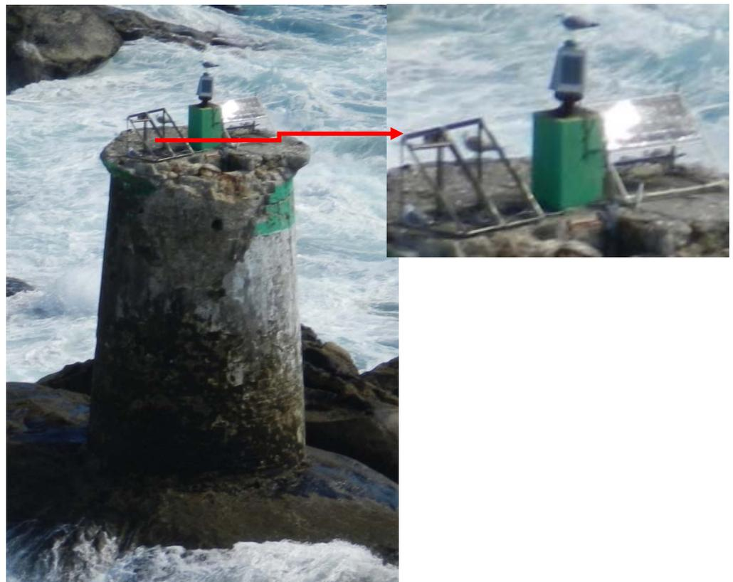
***Figure 2 Northwest of Spain – Galicia coast – Structure and solar panels damages***
