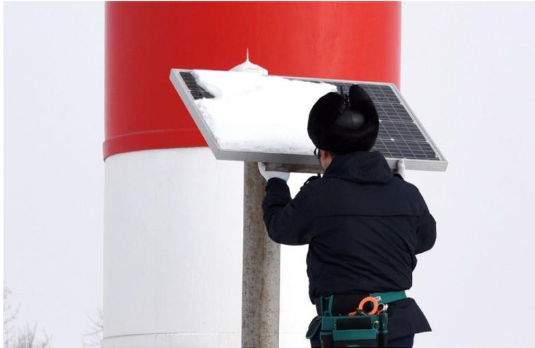
Figure 16 Heavy snow deposits on a solar module in China
