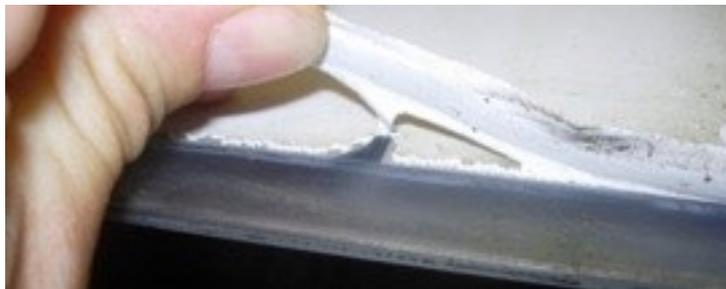
Figure 33 Examples of sealant failure.
