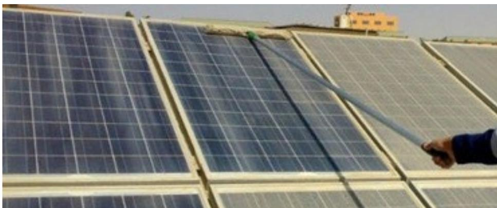
Figure 18 An example of heavy dust deposit
