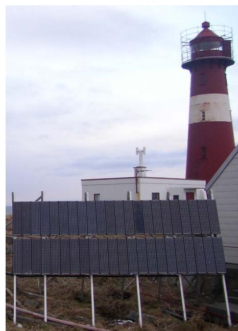
**Figure 2** *Grasøyane lighthouse solar array*
