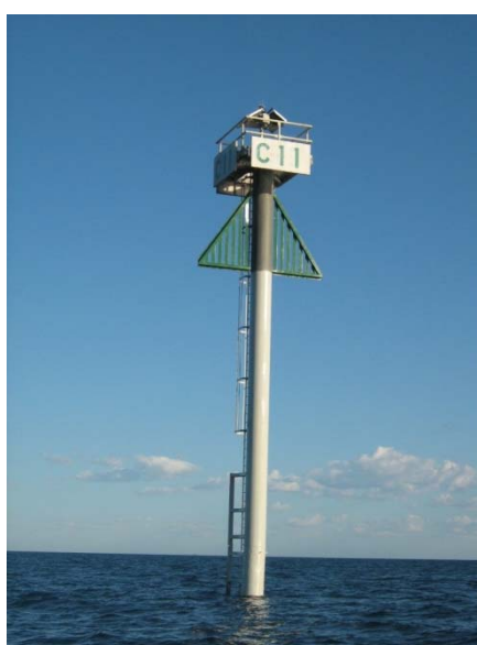
Figure 37 Examples of a fixed structure daymark with unidirectional wings
