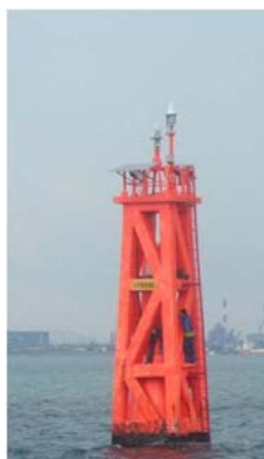
Figure 31 Supporting structure used as a daymark
